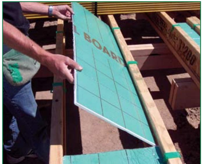
FOILBOARD<sup>®</sup> INSULATION PANEL is being used in conjunction with the FOILBOARD<sup>®</sup> FLOOR SADDLE during the construction process. Note the ease of application.
