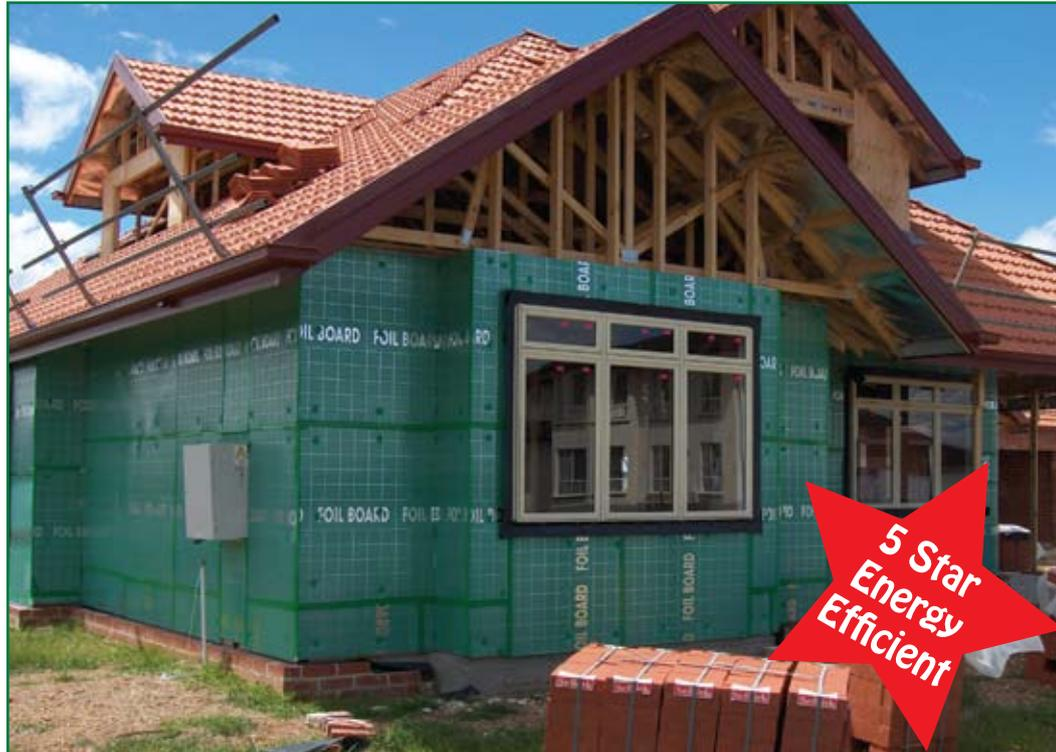
SUPER 15 FOILBOARD<sup>®</sup> INSULATION PANEL has been used on 2.7m walls in Sandringham to achieve an R2.2 rating by a Melbourne project builder. This one insulation product provides a weather proof shield and can slash construction time by up to two weeks. Internal trades go ahead immediately without waiting for brickwork.
