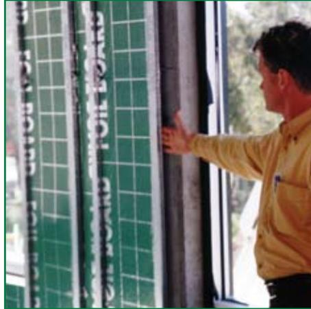
MOTOROLA OFFICE BUILDING - Here we demonstrate how FOILBOARD<sup>®</sup> INSULATION PANEL is applied to concrete structures using Beta-Fix adjustable clips and standard Rondo firing channel.
